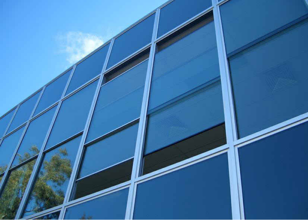
COUNTERBALANCED OPENABLE SASHLESS WINDOWS
